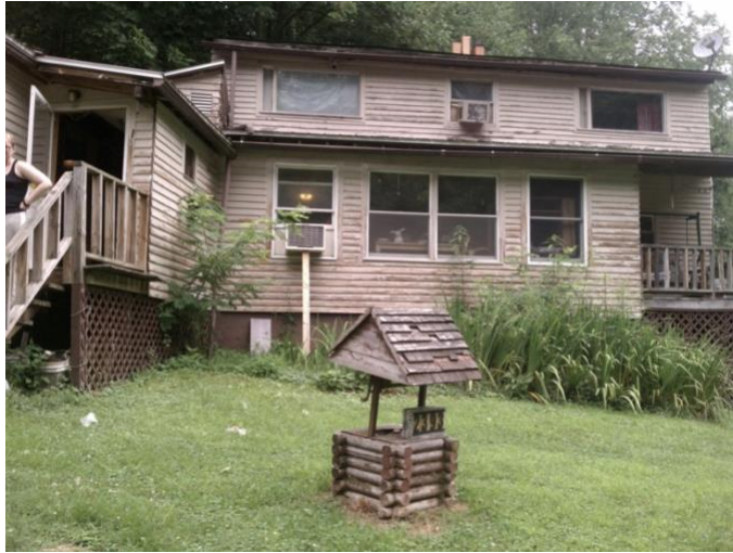
Figure 6: Image of house Ann & Danny built circa 1985
